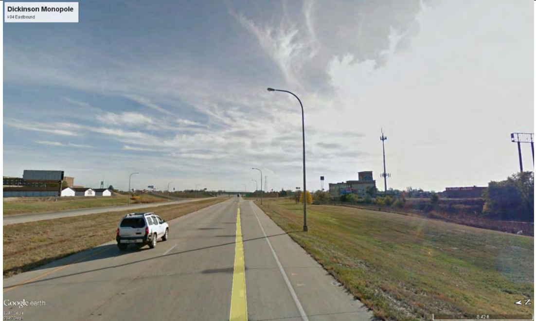
Above: Monopole in Dickinson south of I-94
